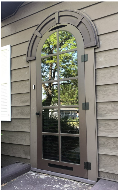
The storm door complete and installed
