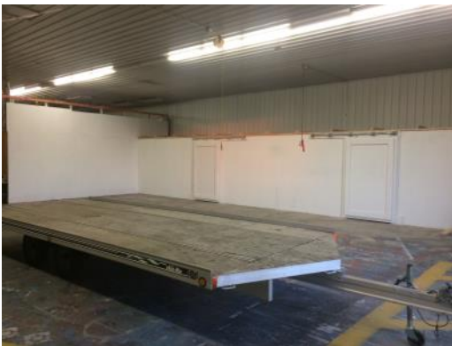
Painting complete and doors hung
